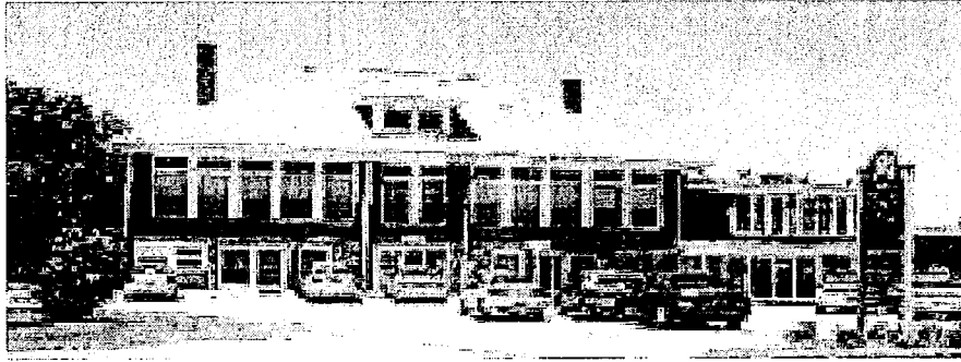
Portsmouth Multi-Purpose Senior Center
