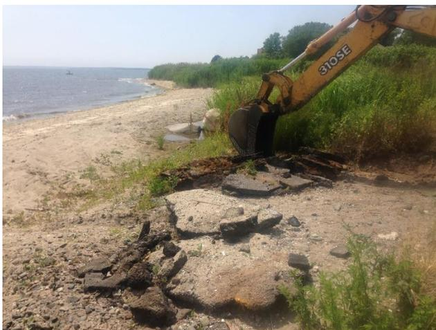
*Eroding pavement at the end of Van Zandt Road in Warwick being removed.*
